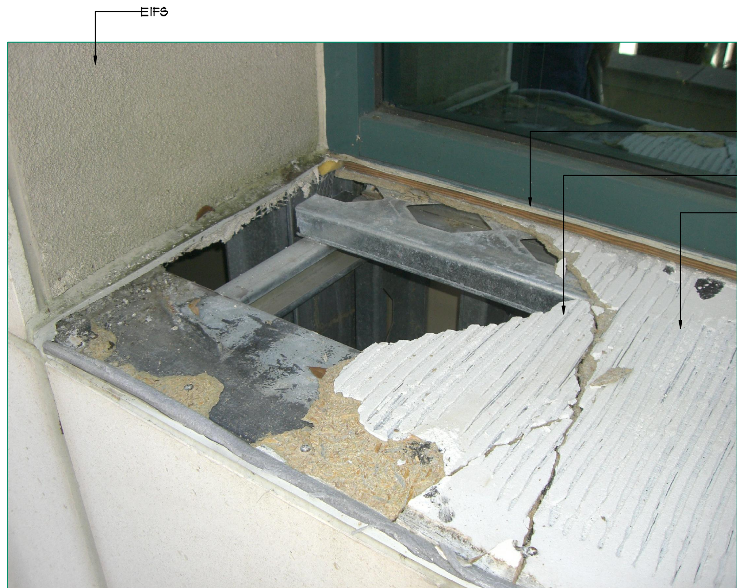
4 EXIST. LEDGER CONDITION 1 of 3 AS-1 NOT TO SCALE
