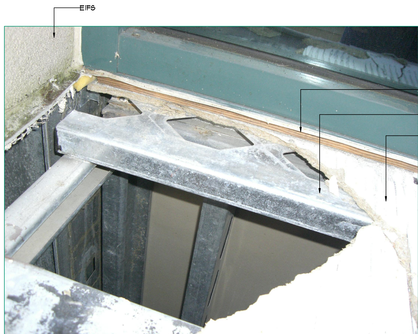
5 EXIST. LEDGER CONDITION 2 of 3 AS-1 NOT TO SCALE
